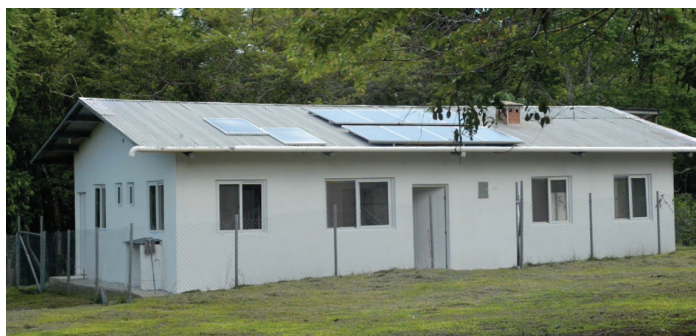
Production plant of coconut oil at Patiño's
